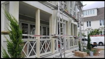
There are multiple examples of spray foam insulation seeping out along the soffit which needs to be cut back and finished as intended.
