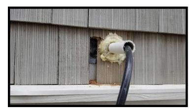
During the inspection, we identified unsealed wall and trim penetrations. As our inspection is not exhaustive, we recommend all wall penetrations, such as window frames, hose bibs, utility boxes, wires and similar points of entry, be reviewed by a specialist and all deficient areas sealed to protect against moisture and insect intrusion.
